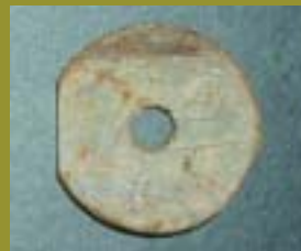
INVERT: SOIL SIDE
