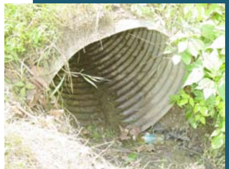
ALT2 Water Side
